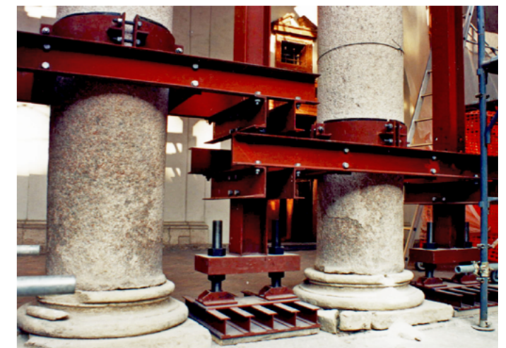
Right down. Replacement of the bases of the columns with a supports system in steel. The basements of the columns were really damaged and the level of degradation could have potential terrible consequences on the stability of the building.
